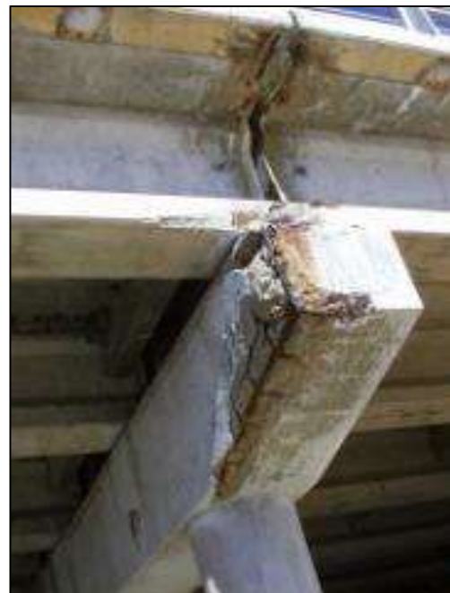
Photo 1 Bridge piers beneath defective joints can be severely affected by de-icing salts washed through with surface run-off water.
