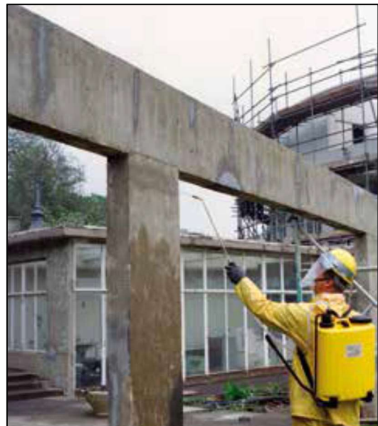
Photo 7 Application of corrosion inhibitors to the concrete
